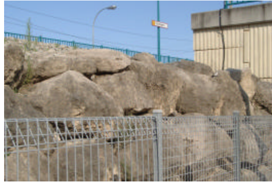
Plate 2 - Limestone blocks at Cannington Railway Station
